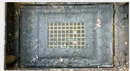
Stays in place. The storm drain insert will not fall into the drain.
