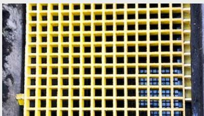
Heavy-duty fiberglass reinforced plastic grating holds the filter in place. Won't corrode or rust.
